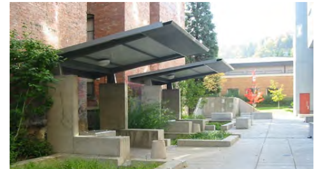
Portland State University, Epler Hall - Rainwater Management
