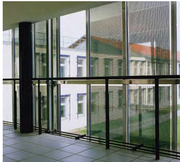
Building Integrated PV
